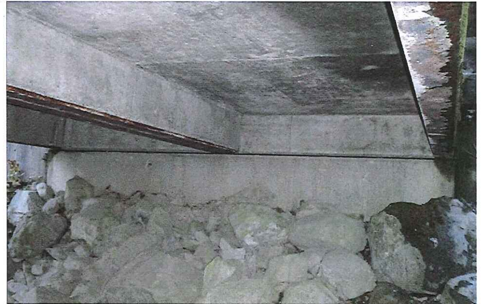
CK2098 Abutment Left Bank
