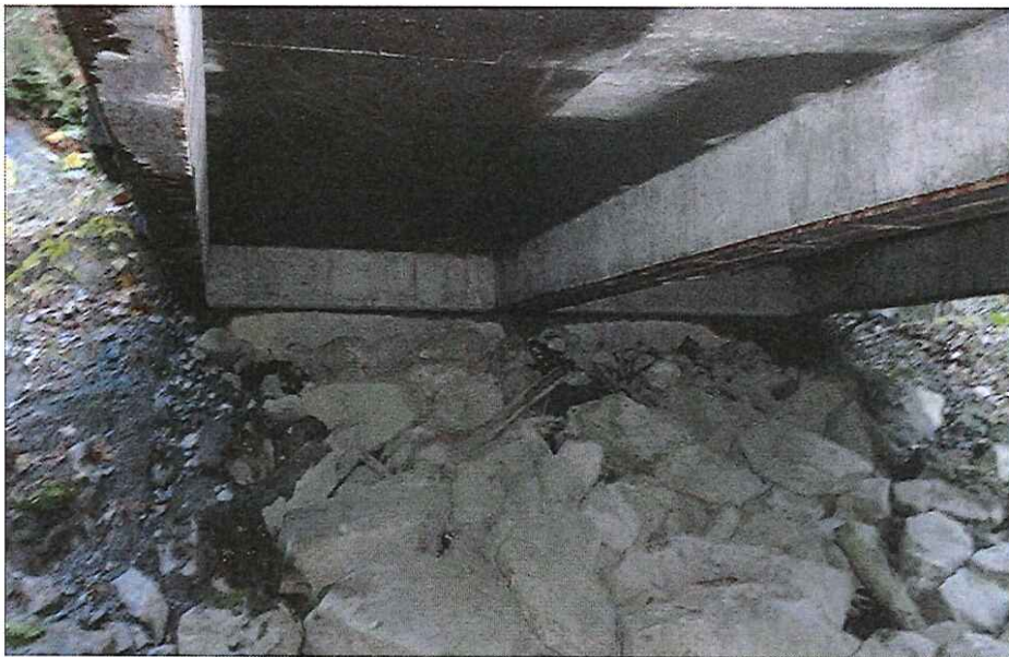
CK2098 Abutment Right Bank
