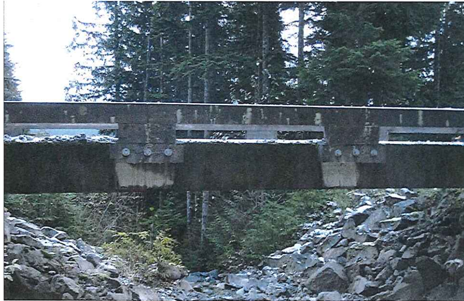
CK2098 Crossing Upstream
