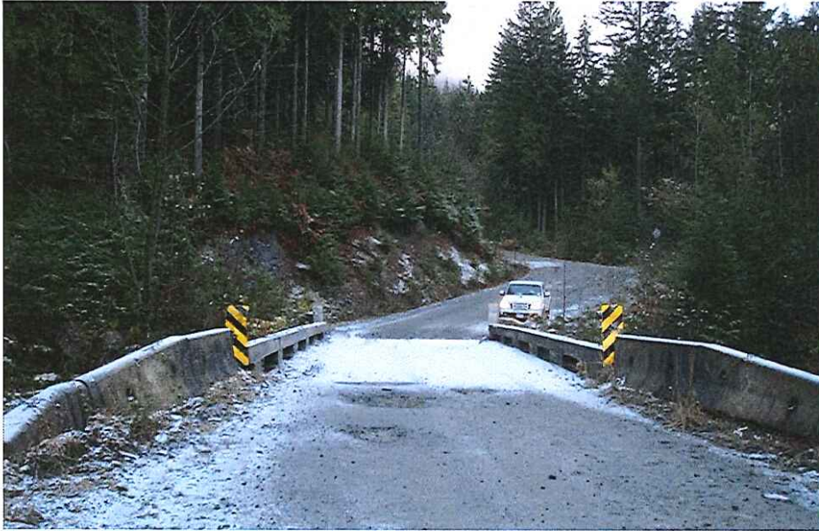
CK2098 Approach Right Bank
