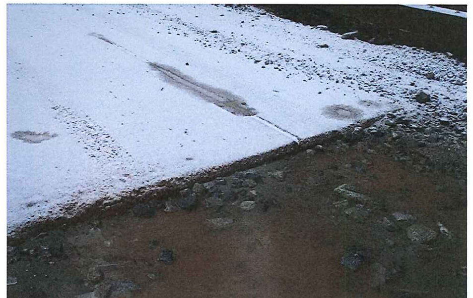
CK2098 Condition of Approaches
